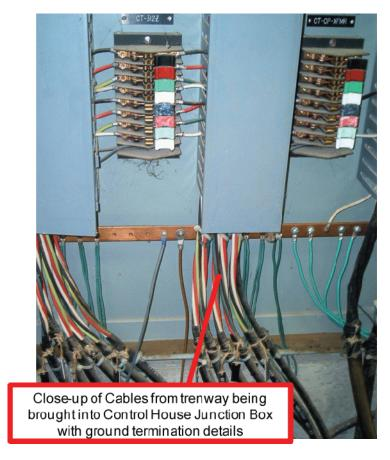
Figure 18: Grounding of control cable shields and j-boxes in control building.<sup>77</sup>
